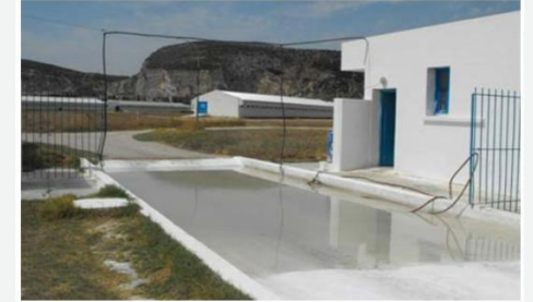
Vehicle disinfection pit
